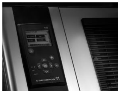
Fig. 28 Grundfos CUE control panel
